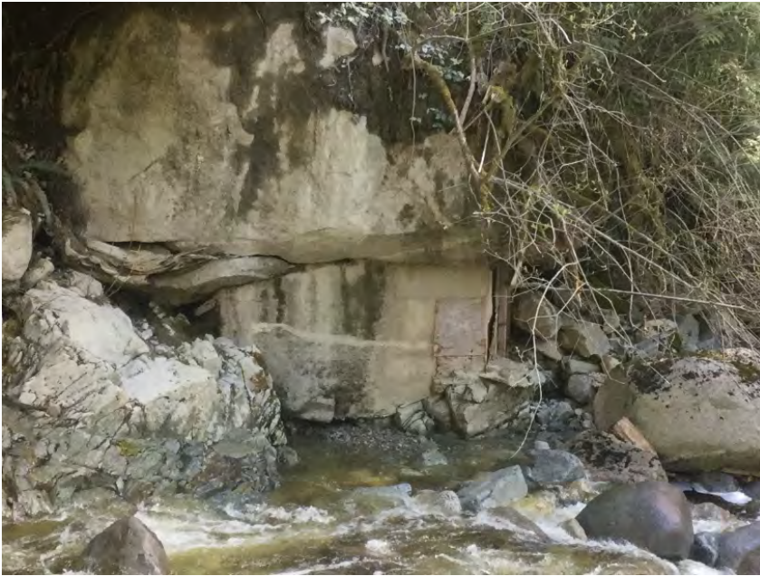
CIP to support large boulder in front of abutment at left bank
