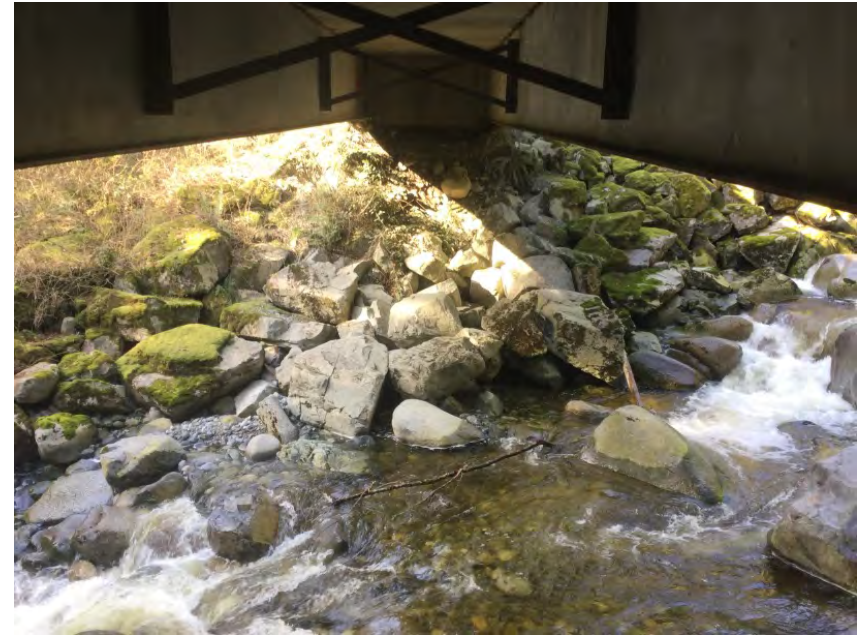
Right Bank Abutment when facing downstream
