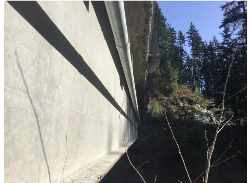
Utility hung fastened to underside of deck
