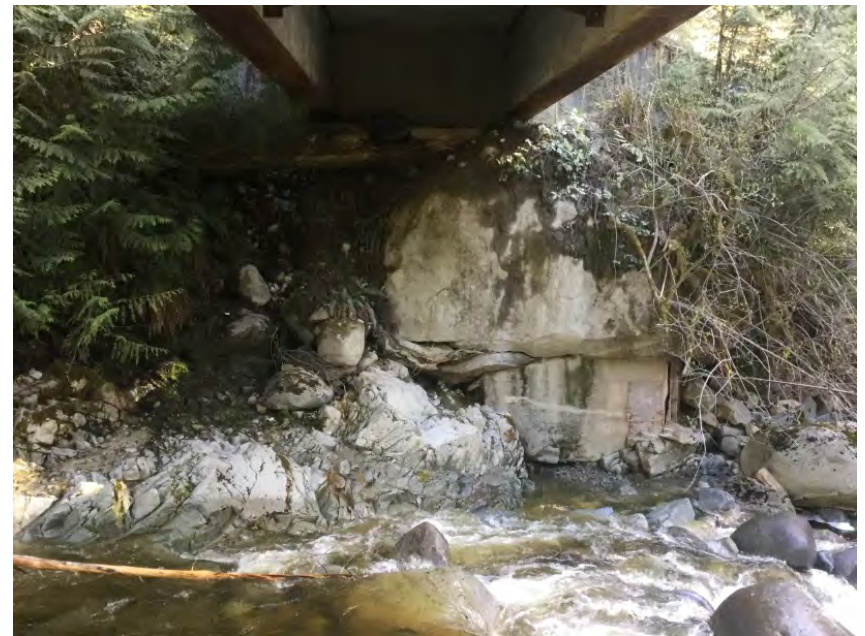
Left Bank Abutment when facing downstream
